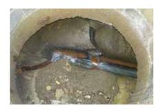
If there are no visible manholes, try visually plotting the likely course of the sewer by studying nearby manholes. Carefully dig a trial hole or trench to locate the pipe.
