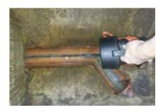
Once you've carefully opened a manhole, you can often work out the direction of flow by turning on a tap or flushing a toilet in your property, then seeing which way the water runs. You might need a torch to help you see. This should help you work out where your property connects in relation to others.
