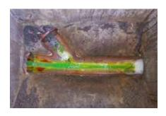
You could try putting dye into your toilet and flushing it, and/or doing the same from a neighbouring property with a different colour dye. This can show where the properties connect into the sewer, as well as the direction of flow.
